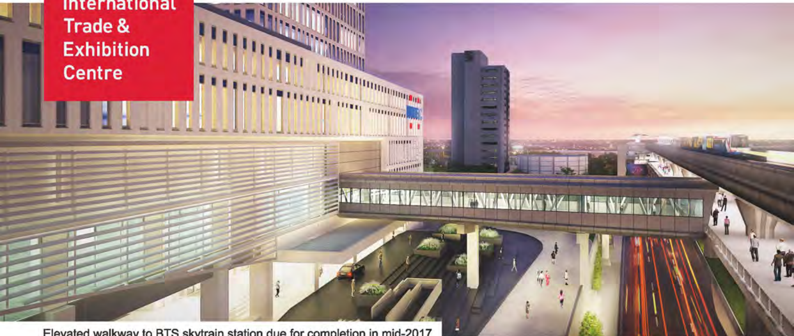
Elevated walkway to BTS skytrain station due for completion in mid-2017
